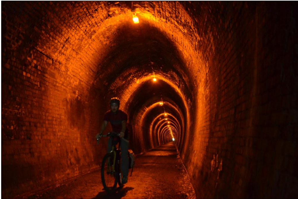
Figure 76: Tunnel on the Hauraki Rail Trail (photo: Jonathan Kennett)
