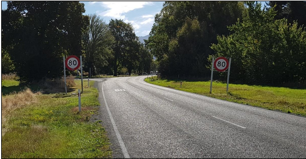
Figure 40: Gated 80 km/h speed limit signs, near Fairlie
