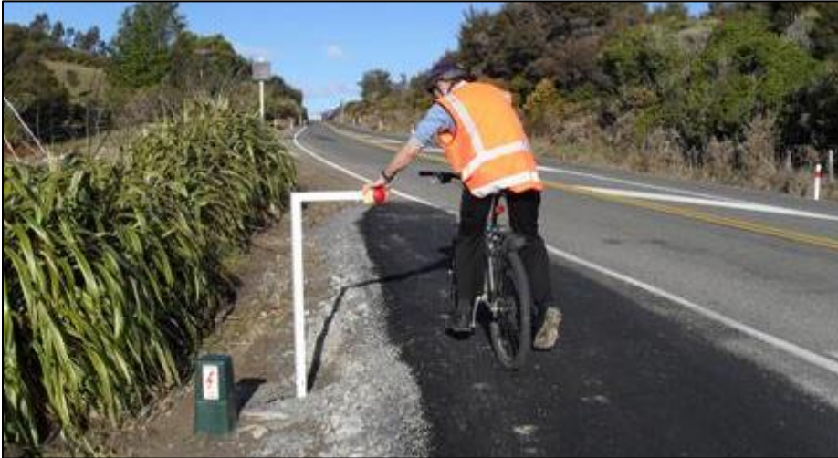
Figure 52: Push button activated warning sign at vertical crest, SH 60 near Nelson (photo: NZTA)
