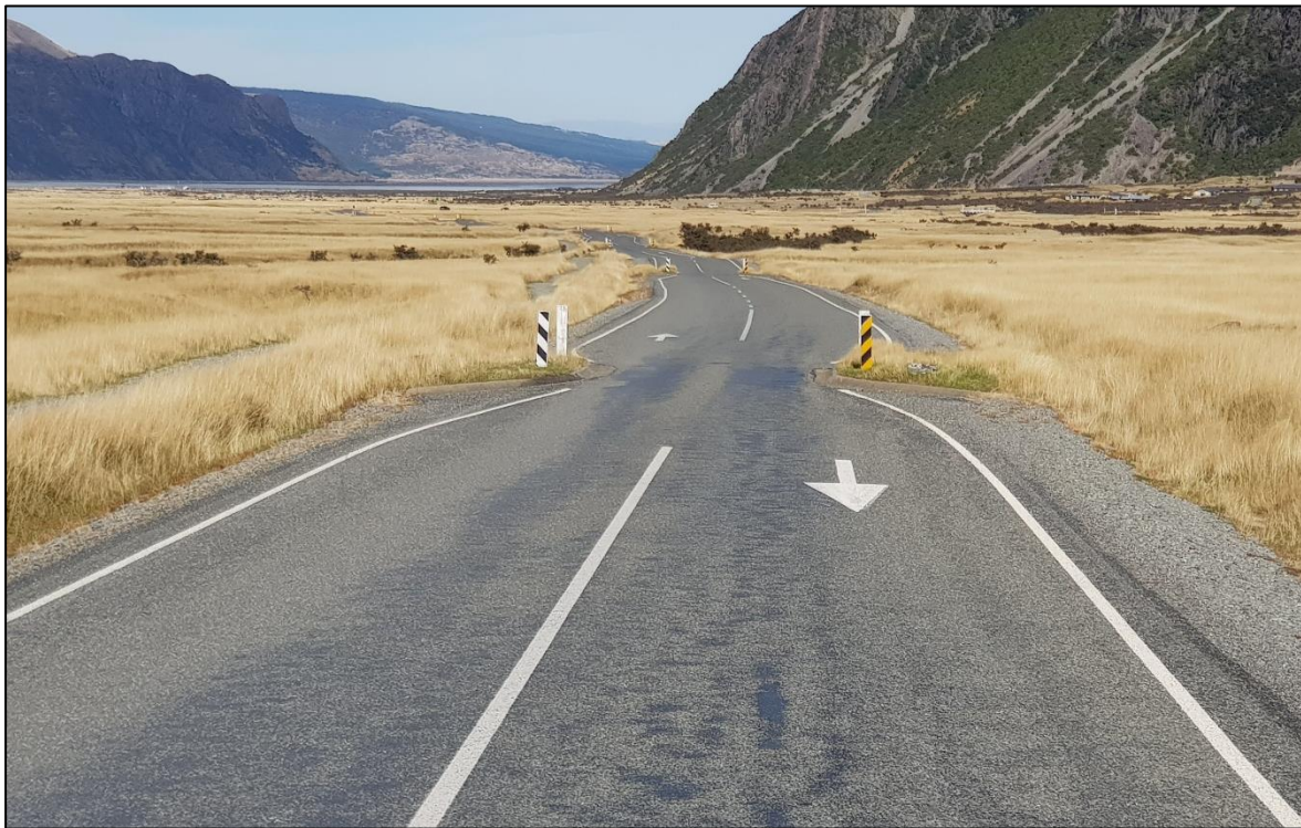
Figure 42: An example of rural traffic calming on a 60 km/h road, Hooker Valley
