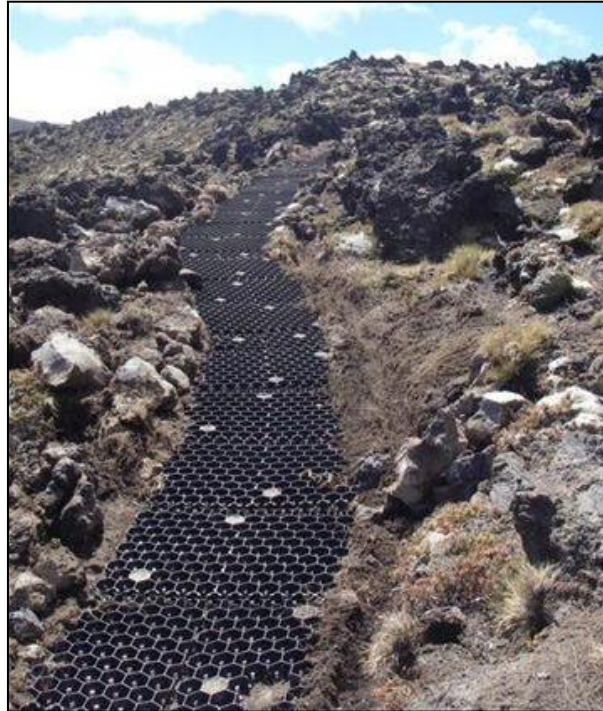
Figure 27: "Geomat" surface stabilisers (prior to having aggregate placed on top), Tongariro National Park (photo: John Bradley)
