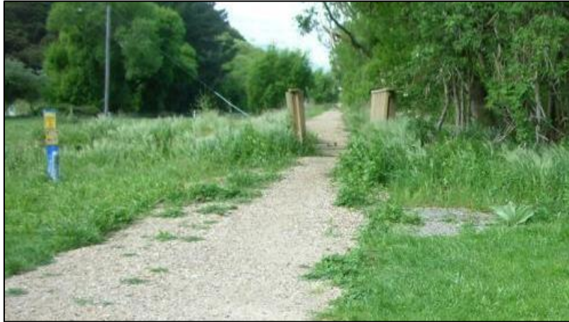
Figure 25: Compacted gravel section of Little River Rail Trail at Catons Bay
