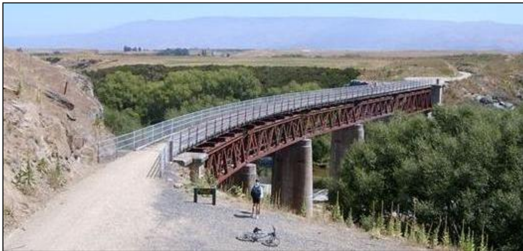
Figure 64: Manuherikia Bridge, Otago Central Rail Trail (photo: DOC)
