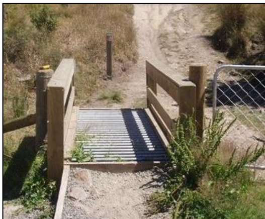
Figure 71: Cattle stop with good alignment, Port Hills (photo: Nick Singleton)
