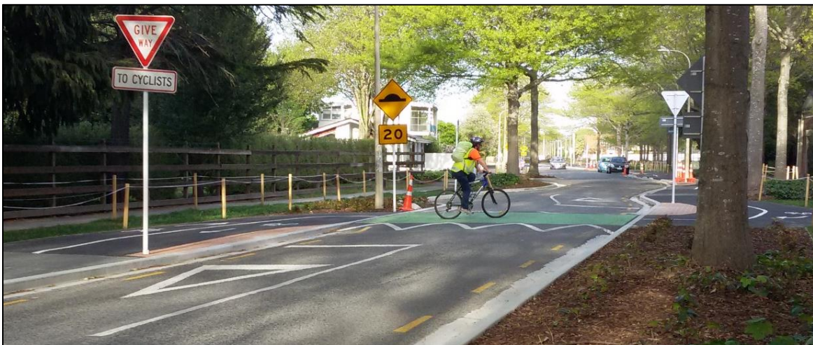
Figure 97: Supplementary “to cyclists” plate on give way sign at midblock priority cycle crossing, Uni-Cycle route, Christchurch
