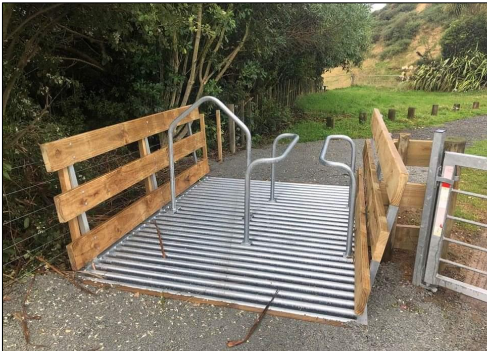
Figure 34: Example of a wheelchair-accessible barrier, Belmont Regional Park (photo: Greater Wellington Regional Council)
