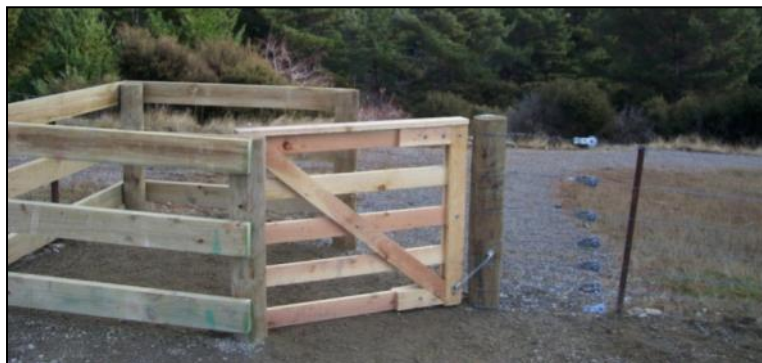
Figure 74: Kissing gate: Hawea Track (since removed); very difficult for tandems, trikes, cargo bikes, trailers
