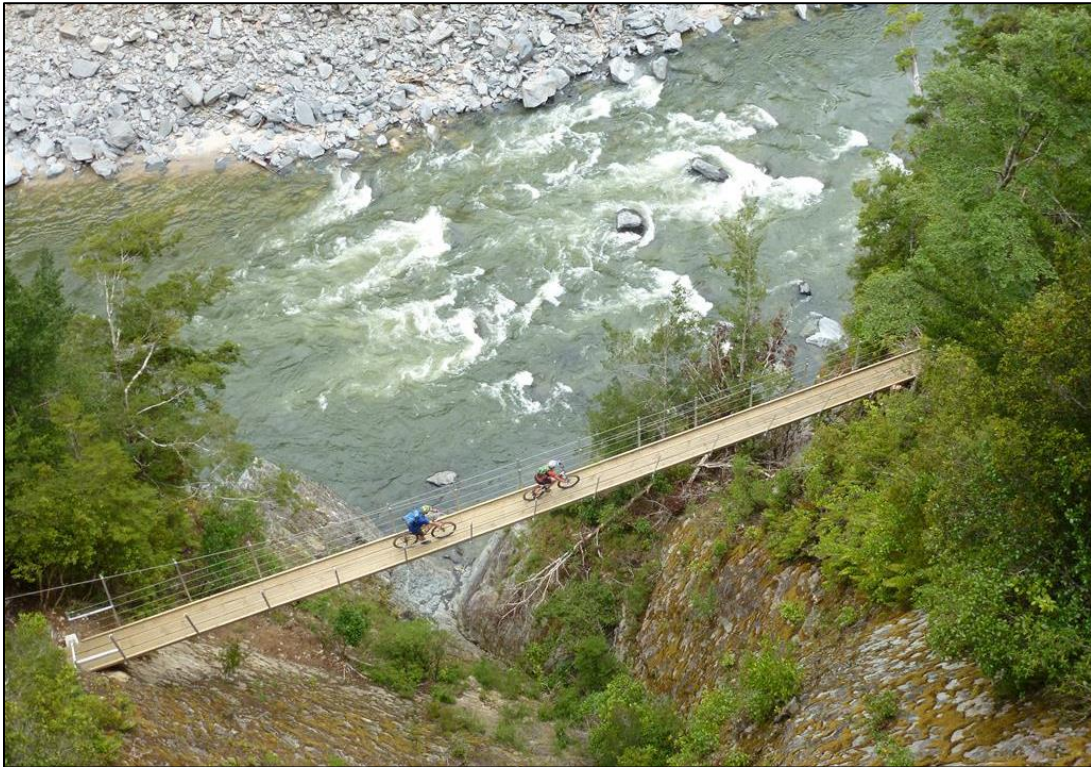
Figure 66: Suspension bridge on the Old Ghost Road (photo: Jonathan Kennett)
