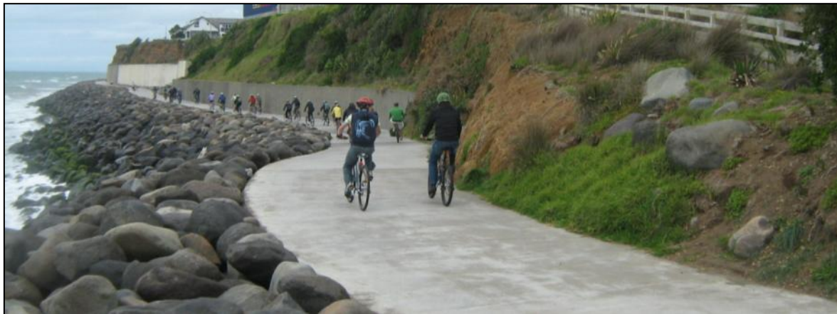
Figure 12: Off-road trail separate from roads – New Plymouth
